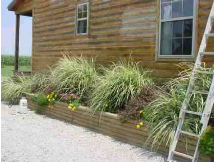
Figure 2.4 Elevated Neosho County Home
