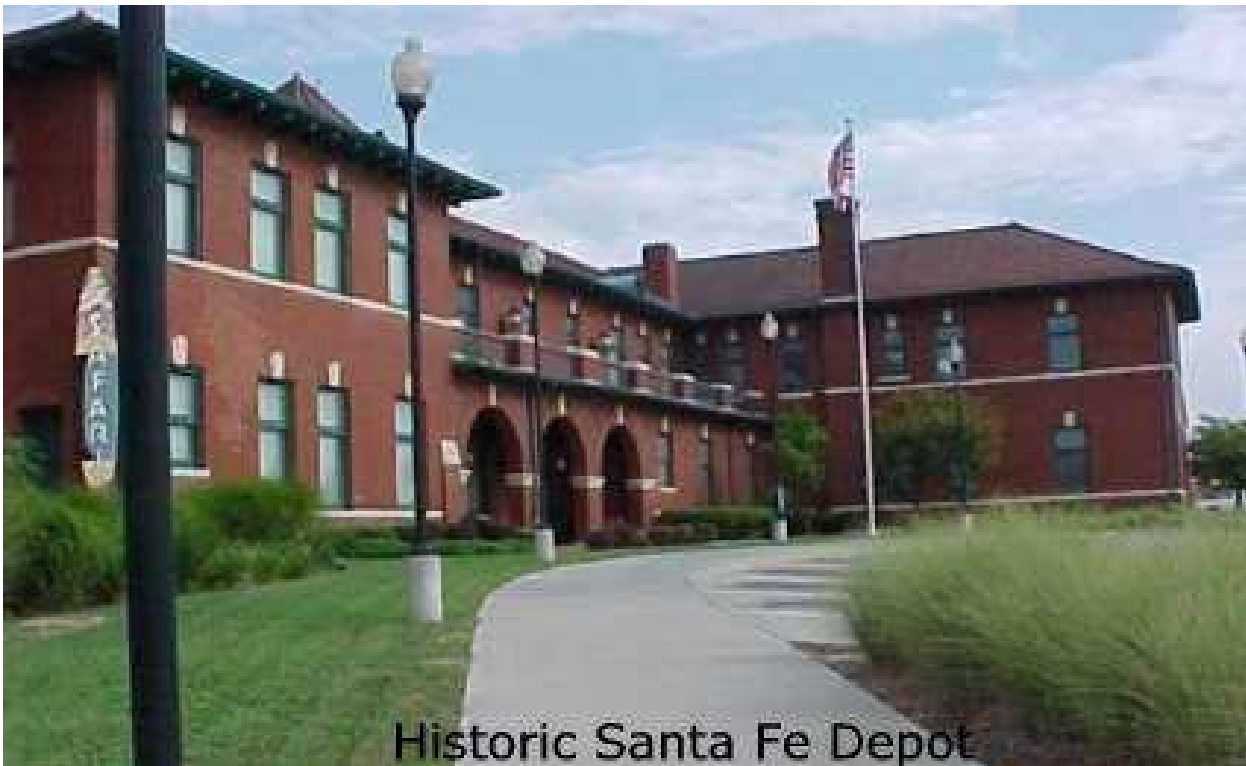
Figure 2.5 Historic Santa Fe Depot
